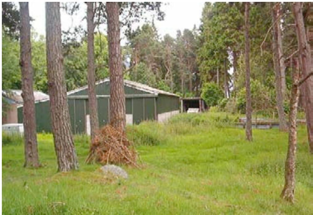
Fig. 8. Site and existing buildings looking south
